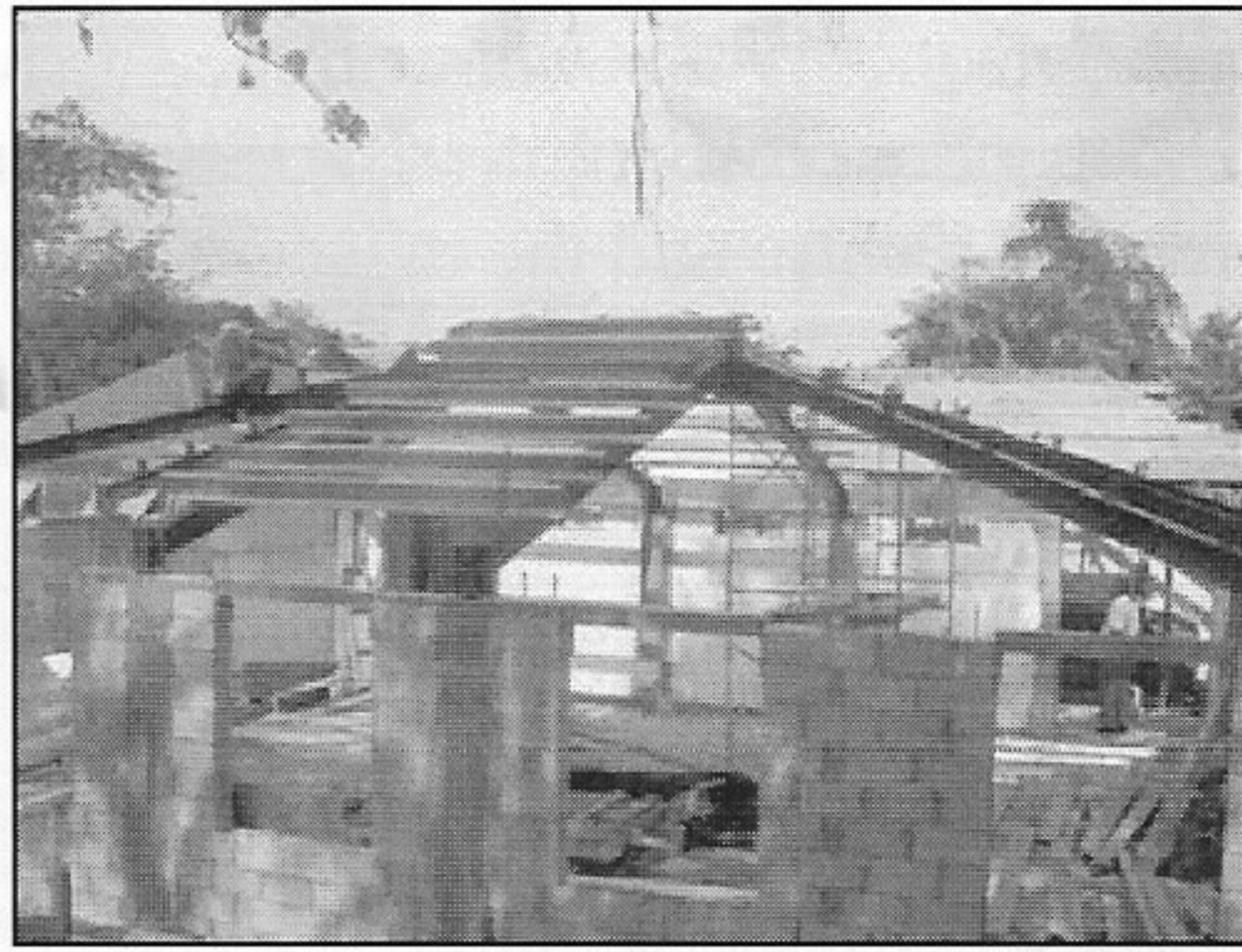
Construction of the new African Gallery
